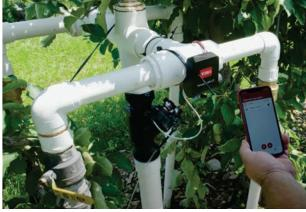
All controllers are connected via Bluetooth on your phone or tablet. This allows you to quickly adjust irrigation schedules or look at performance data in the field. All cluster programs are adjusted via the web-based platform.
